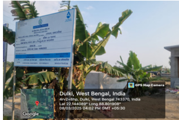
Figure 5: Condition of the JJM project in the Dulki Village
